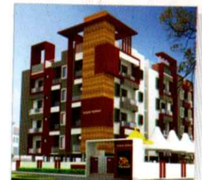
IYYANGARAN APARTMENTS (40 Deluxe flats) Brindavan Road, Fairlands, Salem
